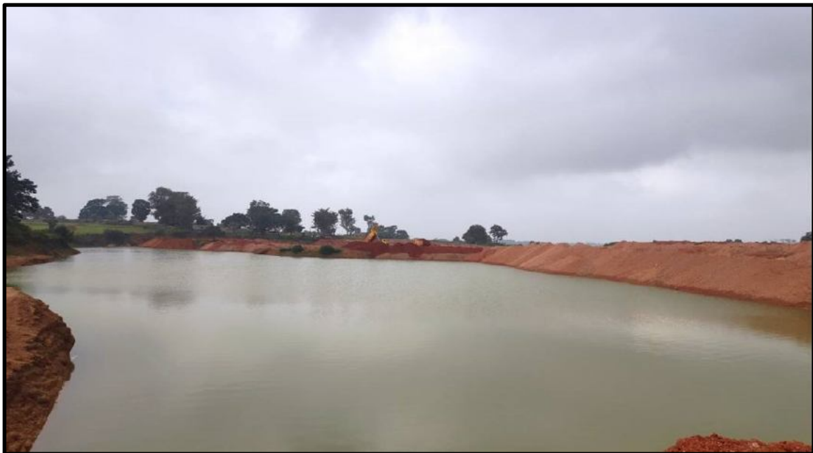
(Rainwater harvesting pond)
