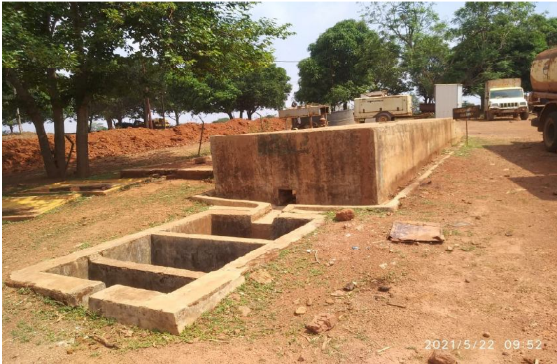
(Washing Ramp and Oil and grease trap)
