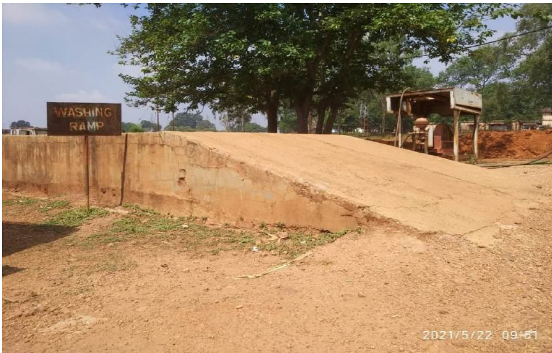
(Washing platform and oil & grease trap)
