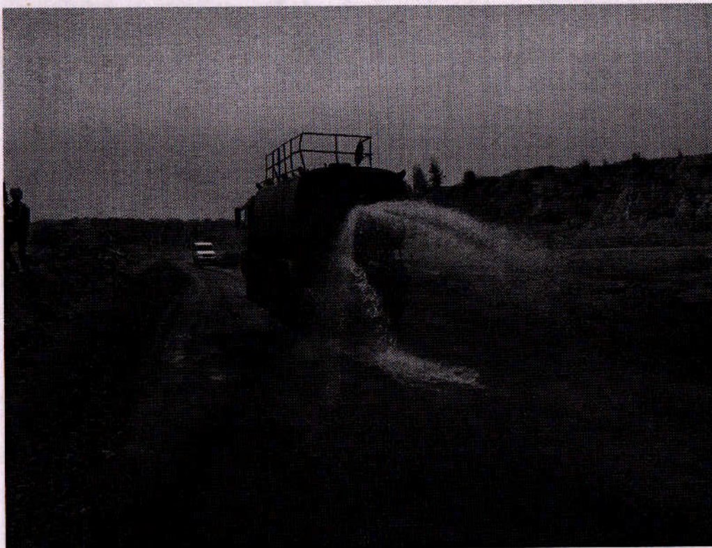
Figure 4: Water sprinkling by truck for Dust Suppression
