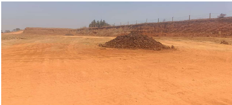
Land preparation for reclamation
