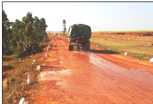
Water Sprinkling in the Haul Road
