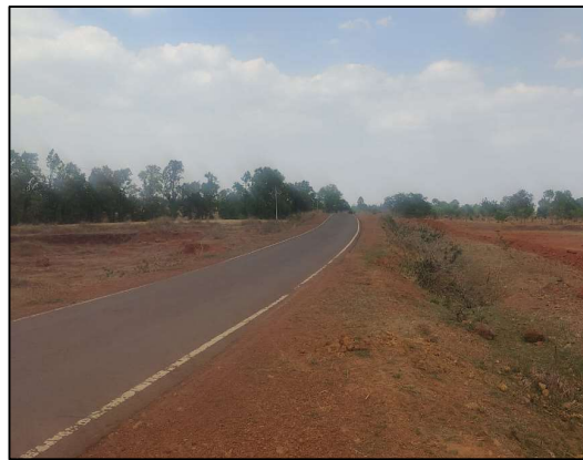
Black top access road to the mines
