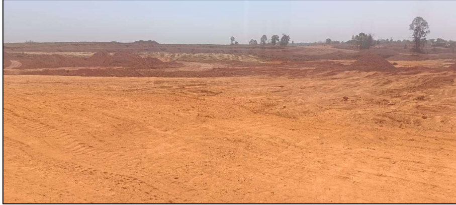
Top Soil Spreading for Backfilling
