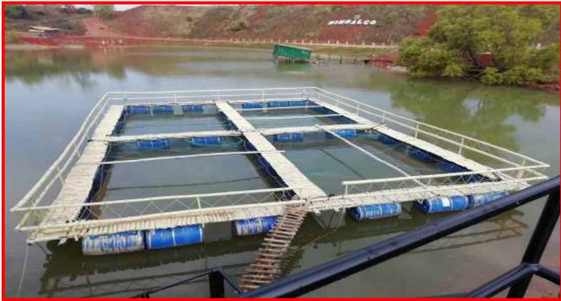
Rainwater Harvesting Pond
