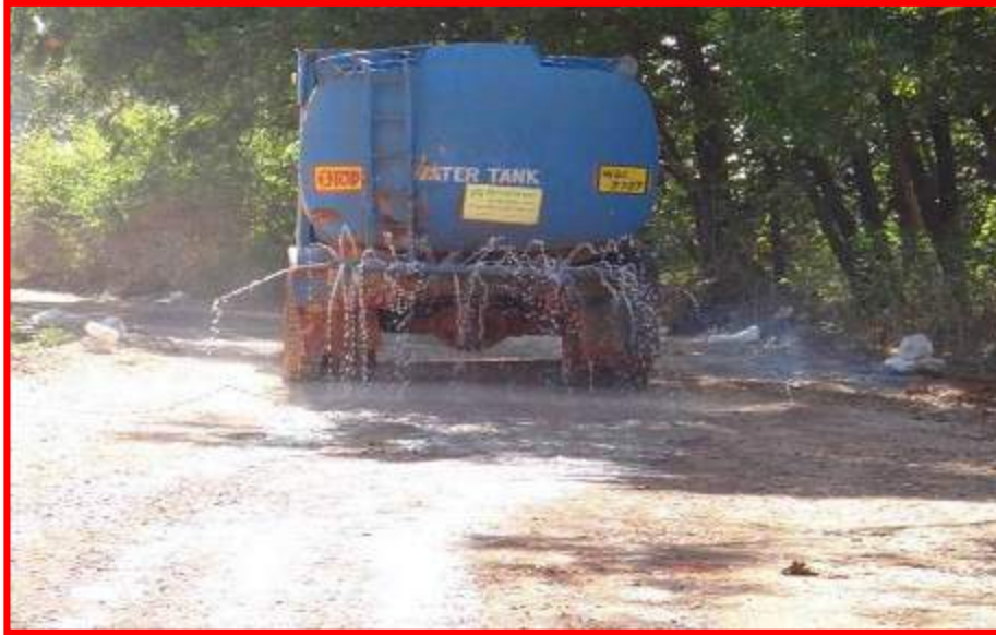
Water sprinkling on road
