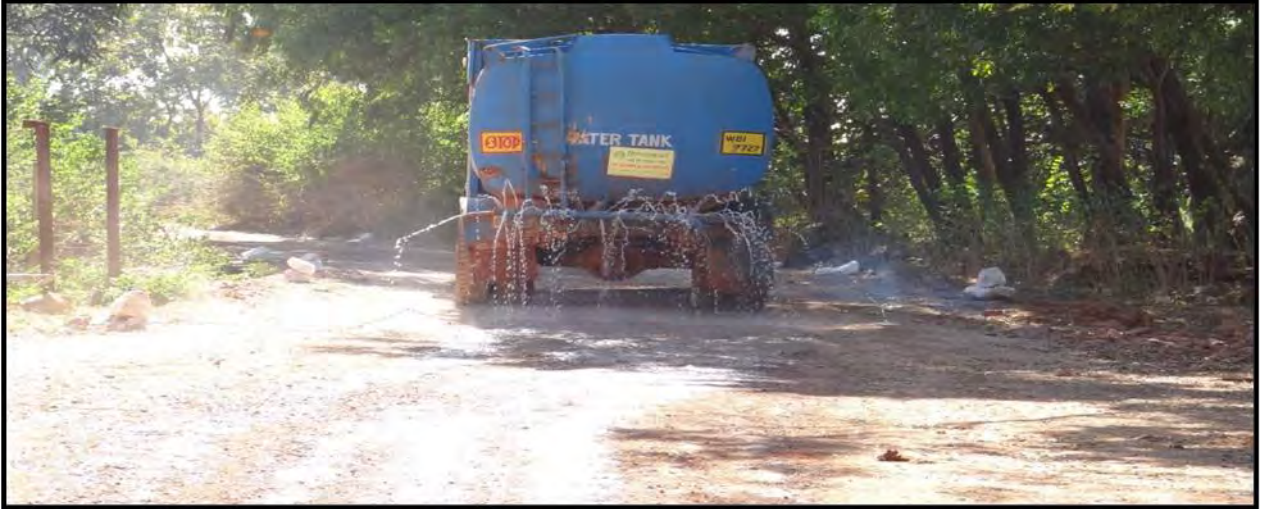
Water Sprinkling at Bagru Mines
