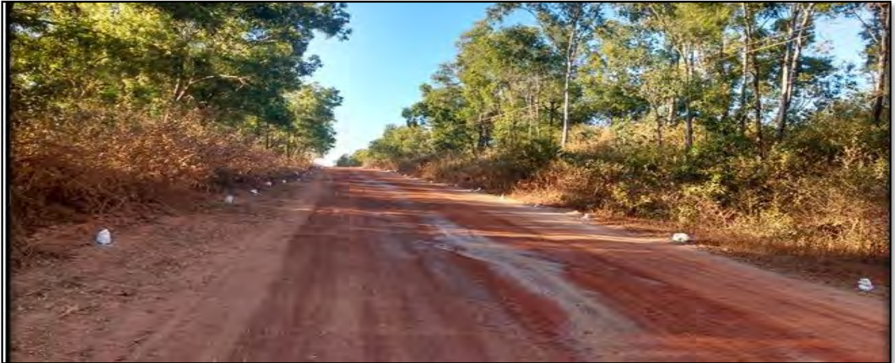
Green Belt Development along Road side
