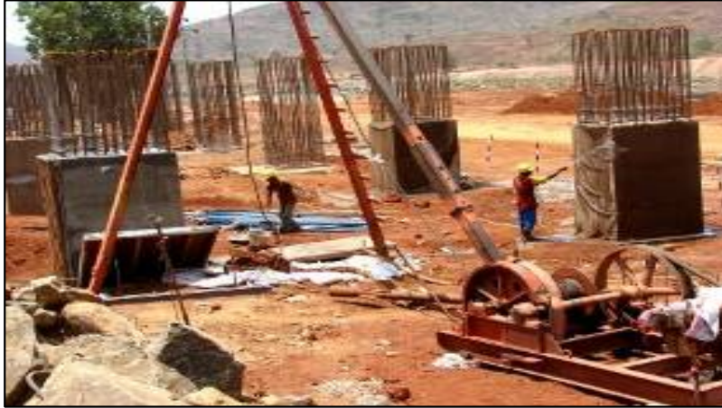
L & T : Piling under progress for civil foundations of pipe racks
