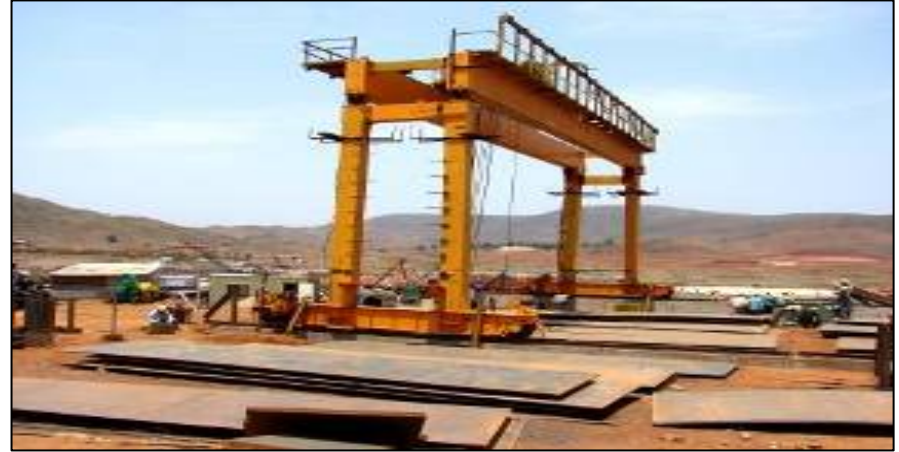
L & T Fabrication Yard : Gantry crane for fabrication – Load test under progress
