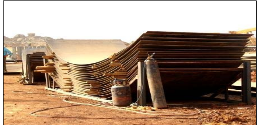
Stock pile of rolled plates for tankages
