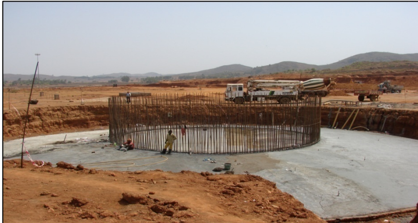
RRCimney for CPP- Raft foundation
