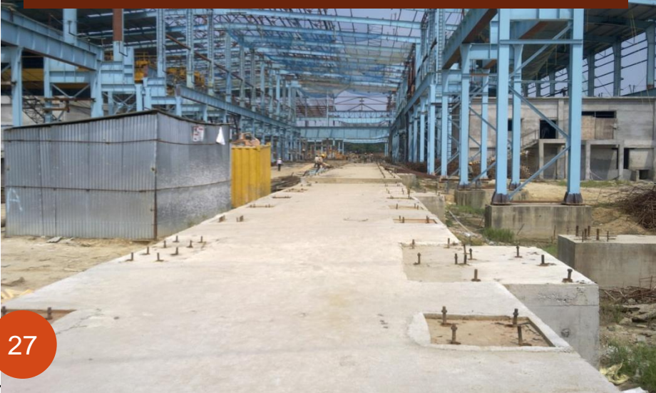
Hot Mill Table Roll Foundation
