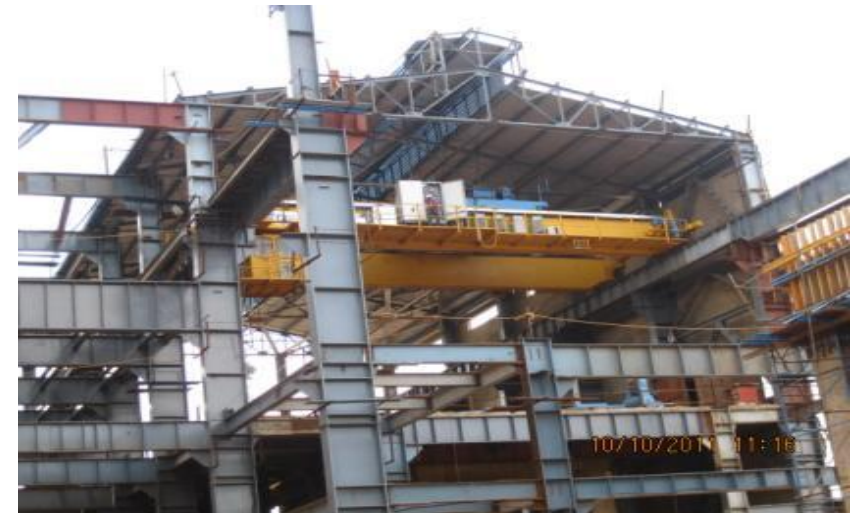
STG1: EOT Crane erection
