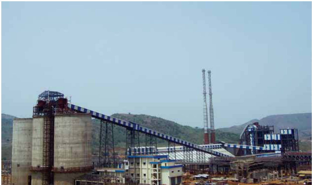
Utkal Alumina International Ltd.
