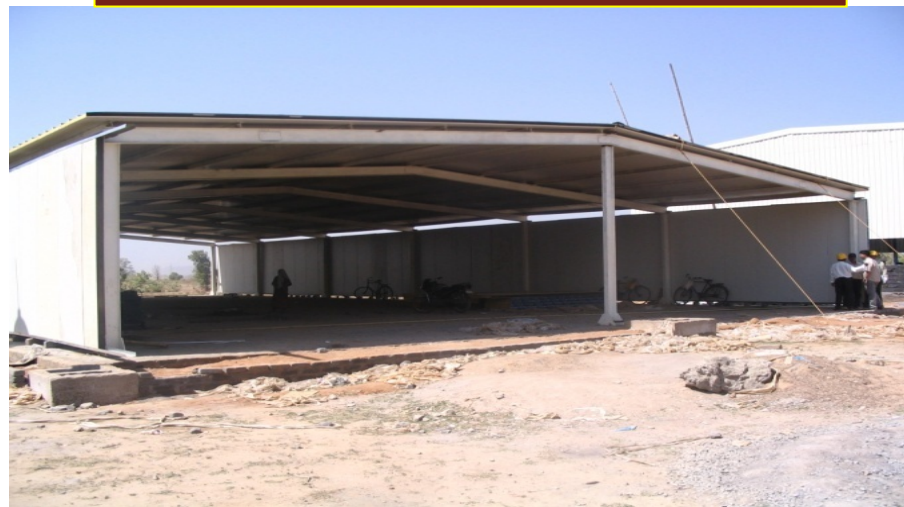
GTC Area Store under construction
