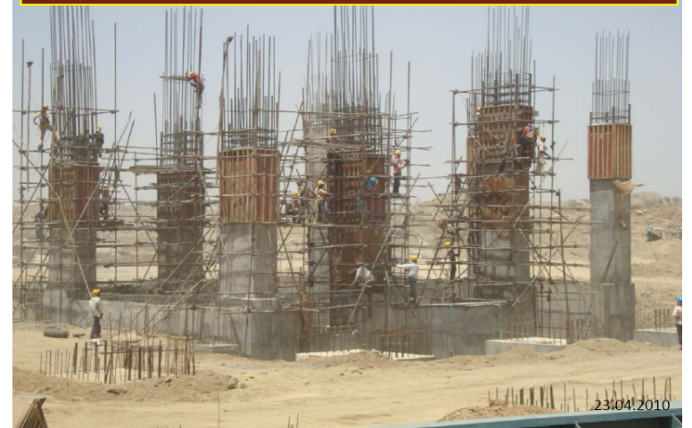
TG#1 RCC Columns: Reinforcement and shuttering in progress
