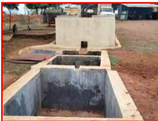
Washing Ramp and Oil and Grease Trap
