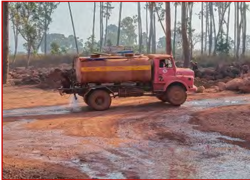
Dust Suppression through water tanker.
