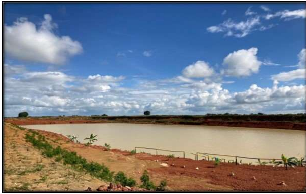
Rain Water Harvesting Pond
