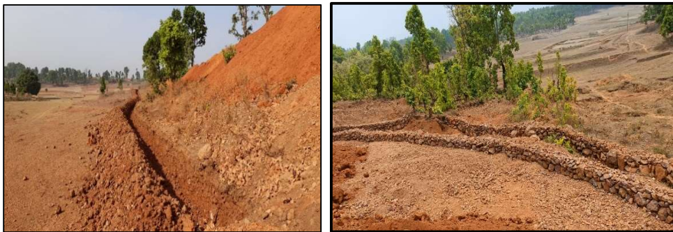
Photographs of garland drains and parapet wall
