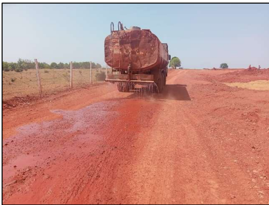
Water Sprinkling in haul road
