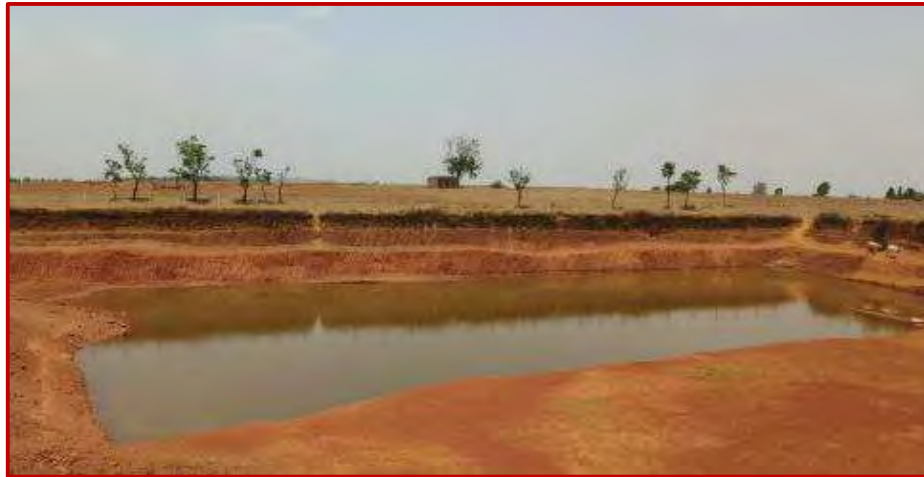
Rainwater Harvesting Pond
