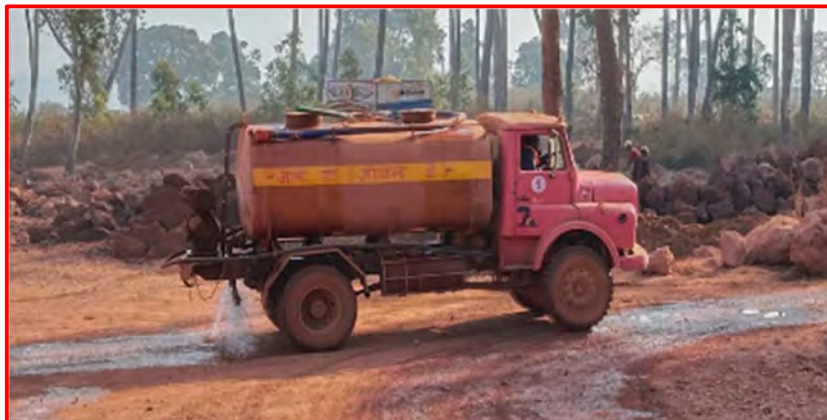
Water sprinkling through tanker.
