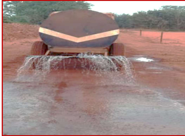
Water sprinkling through tanker.
