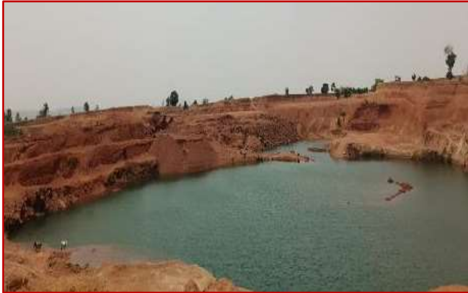
Rainwater Harvesting Pond
