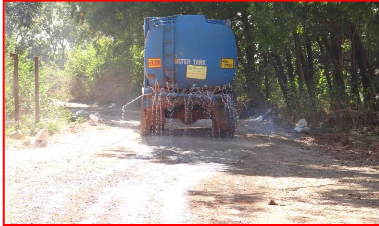
Water Sprinkling on Haul Road
