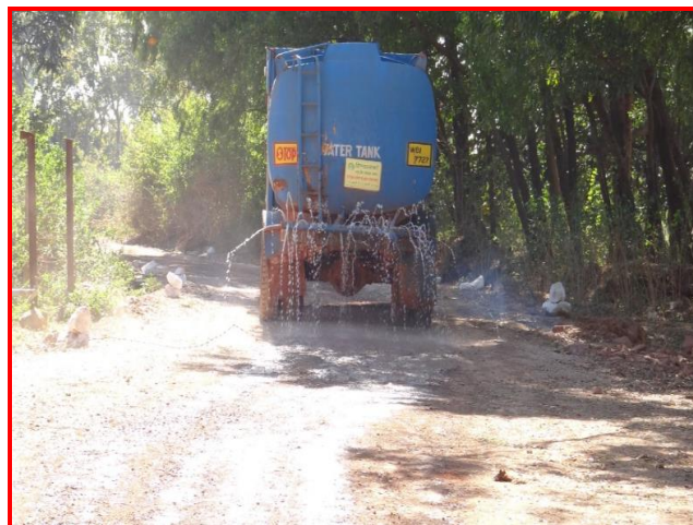
Water Sprinkling on Haul Road
