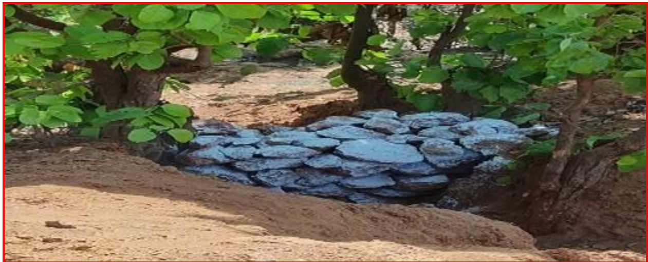
Retaining wall to prevent solid wash-off.
