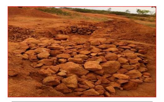
Check drain and Siltation pit around mine pit to prevent runoff.
