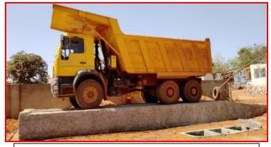
Washing Ramp with Oil and Grease Trap
