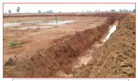
Garland drains around mine pit to prevent runoff.
