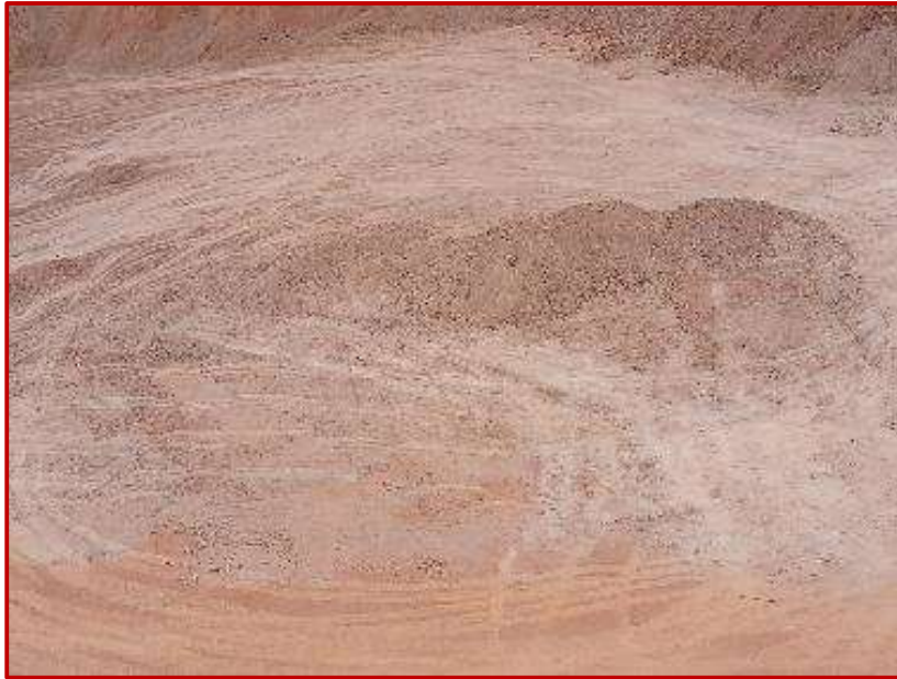
Reclamation of the mined-out
