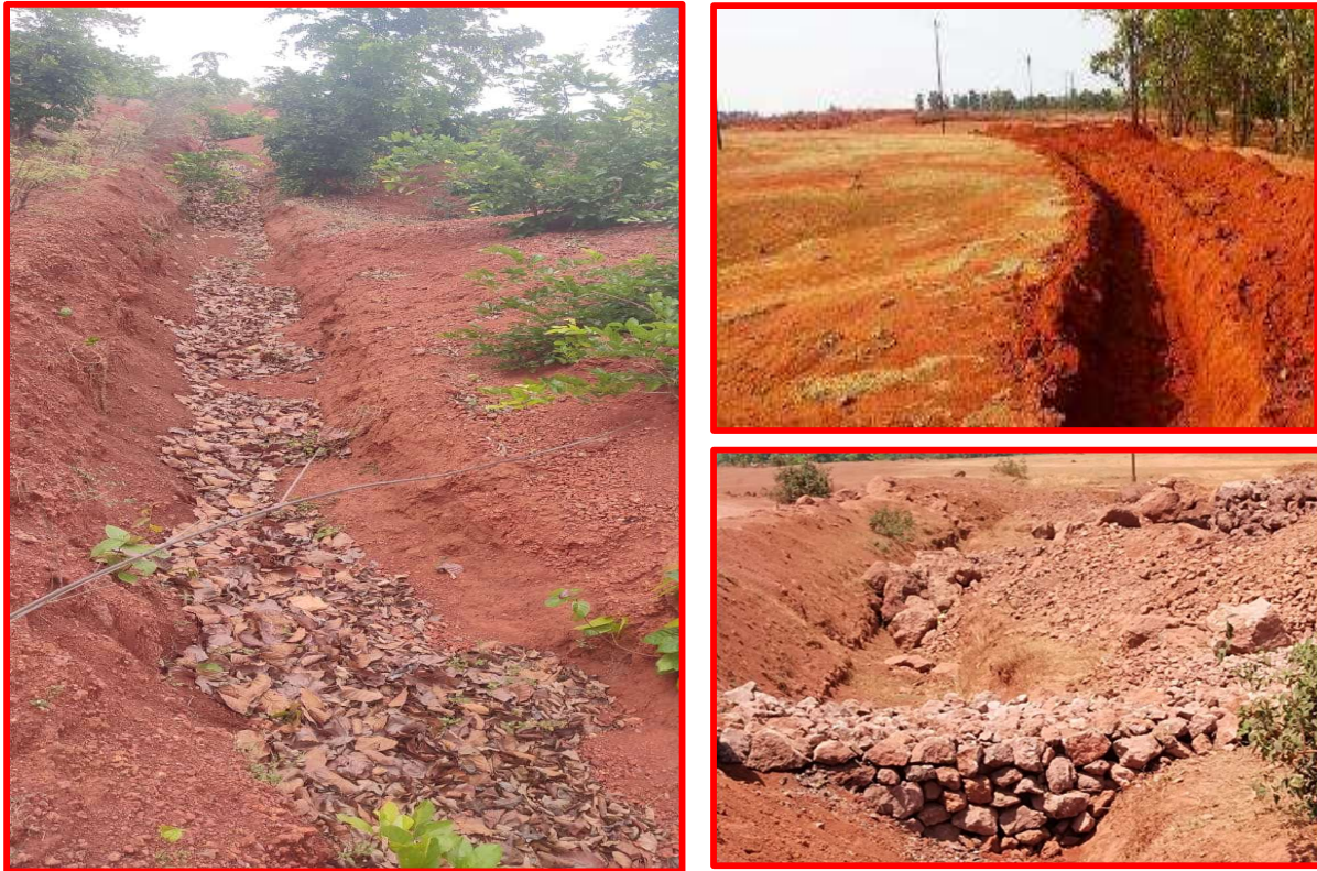
Garland drains & Siltation Pond
