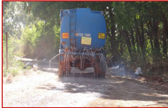
Water sprinkling through tanker.
