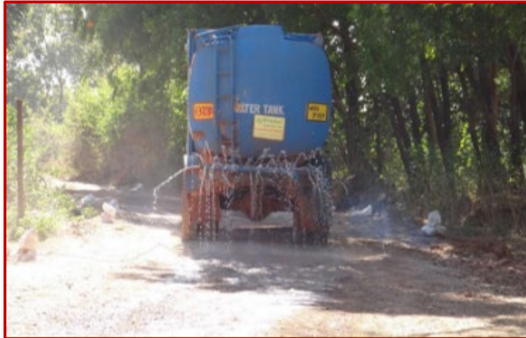
Water sprinkling through tanker.
