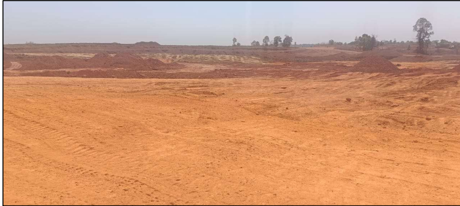
Top Soil Spreading for Backfilling
