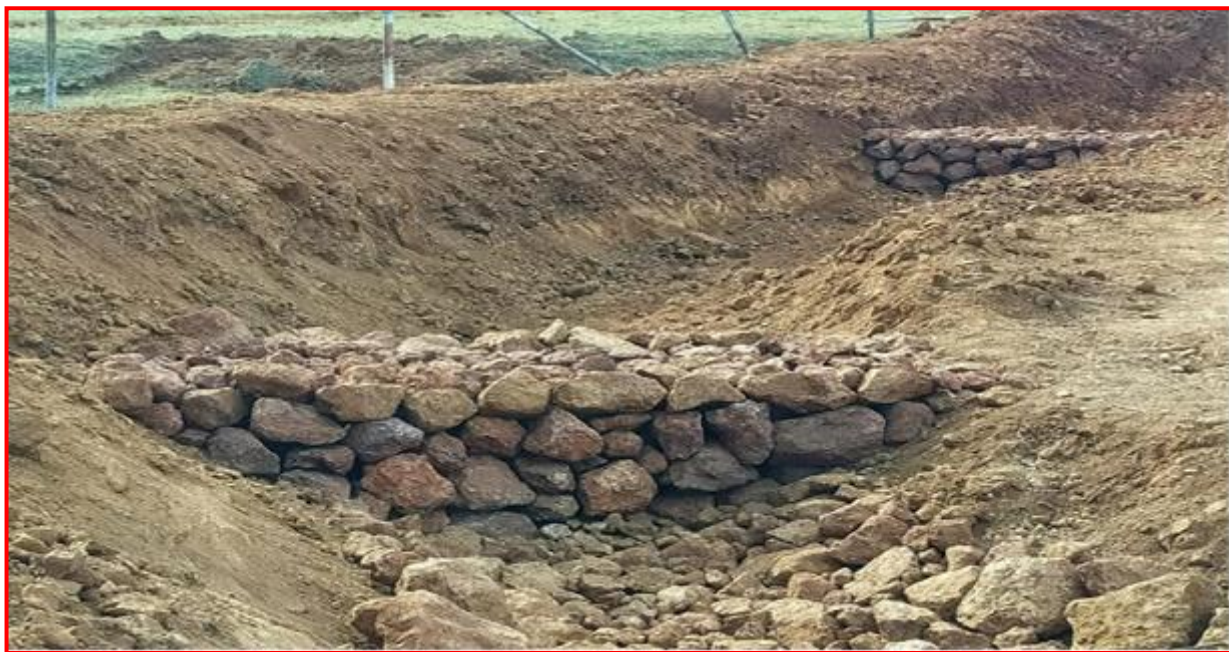
Catch drain Near mine pit.
