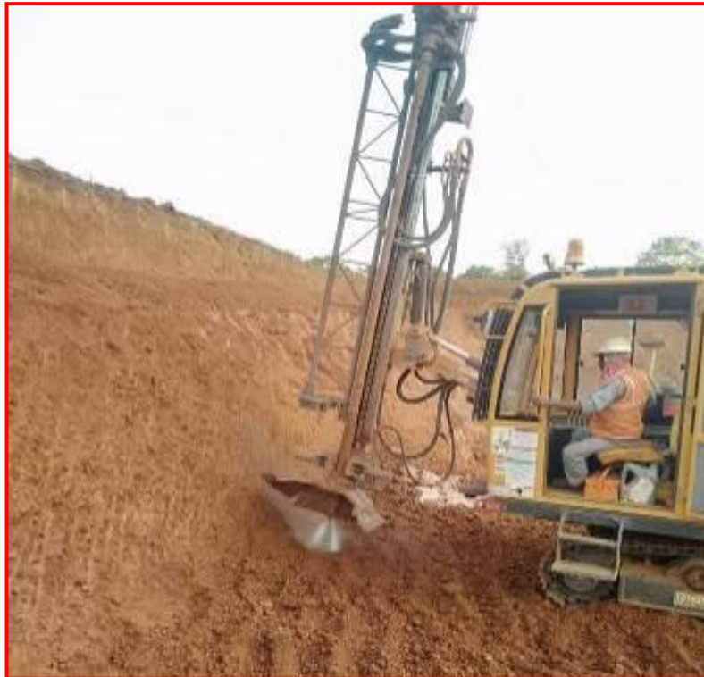
Wet drilling is being carried out.
