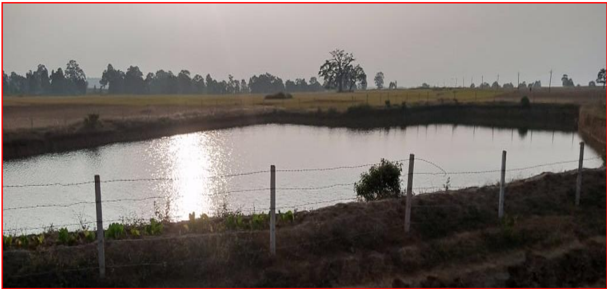
Rainwater Harvesting Pond.
