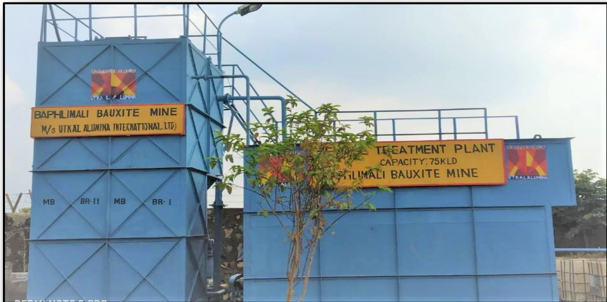
PHOTO 16: Showing 75 KLD Sewage Treatment Plant (STP)
