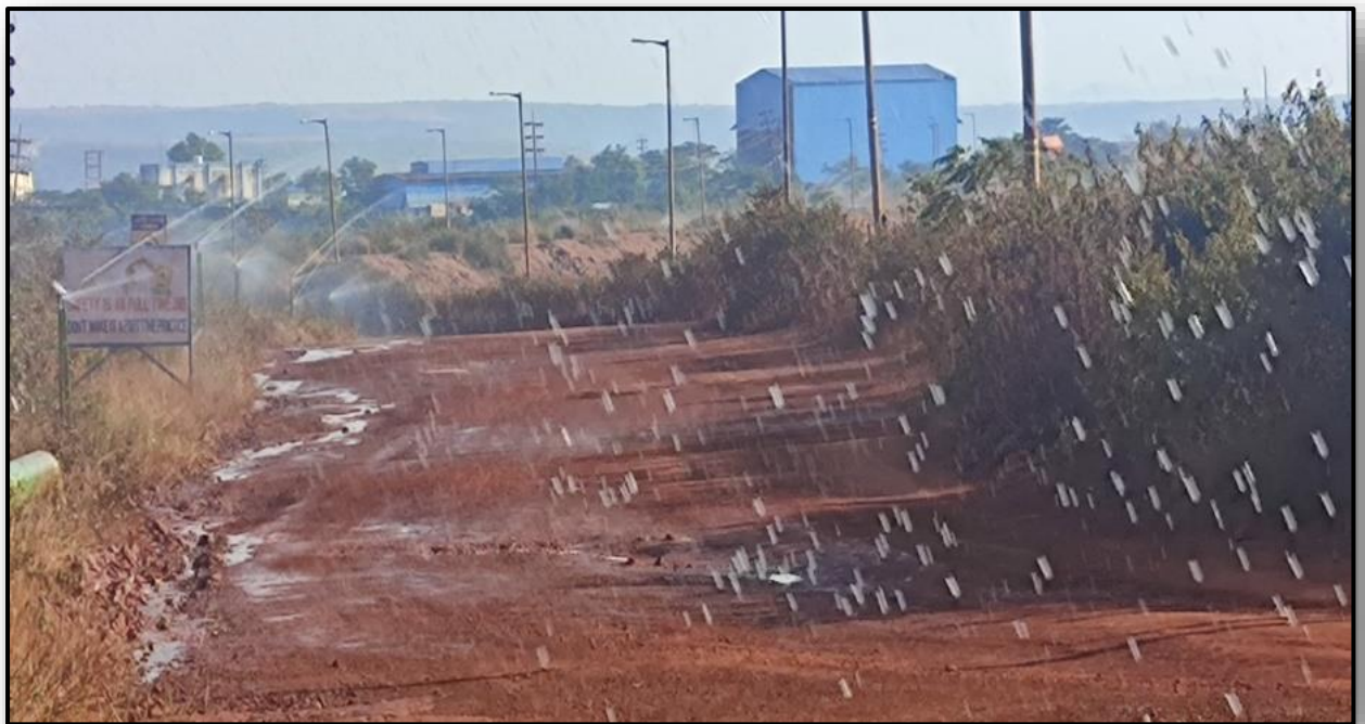
PHOTO 9: Showing Fixed Sprinklers
