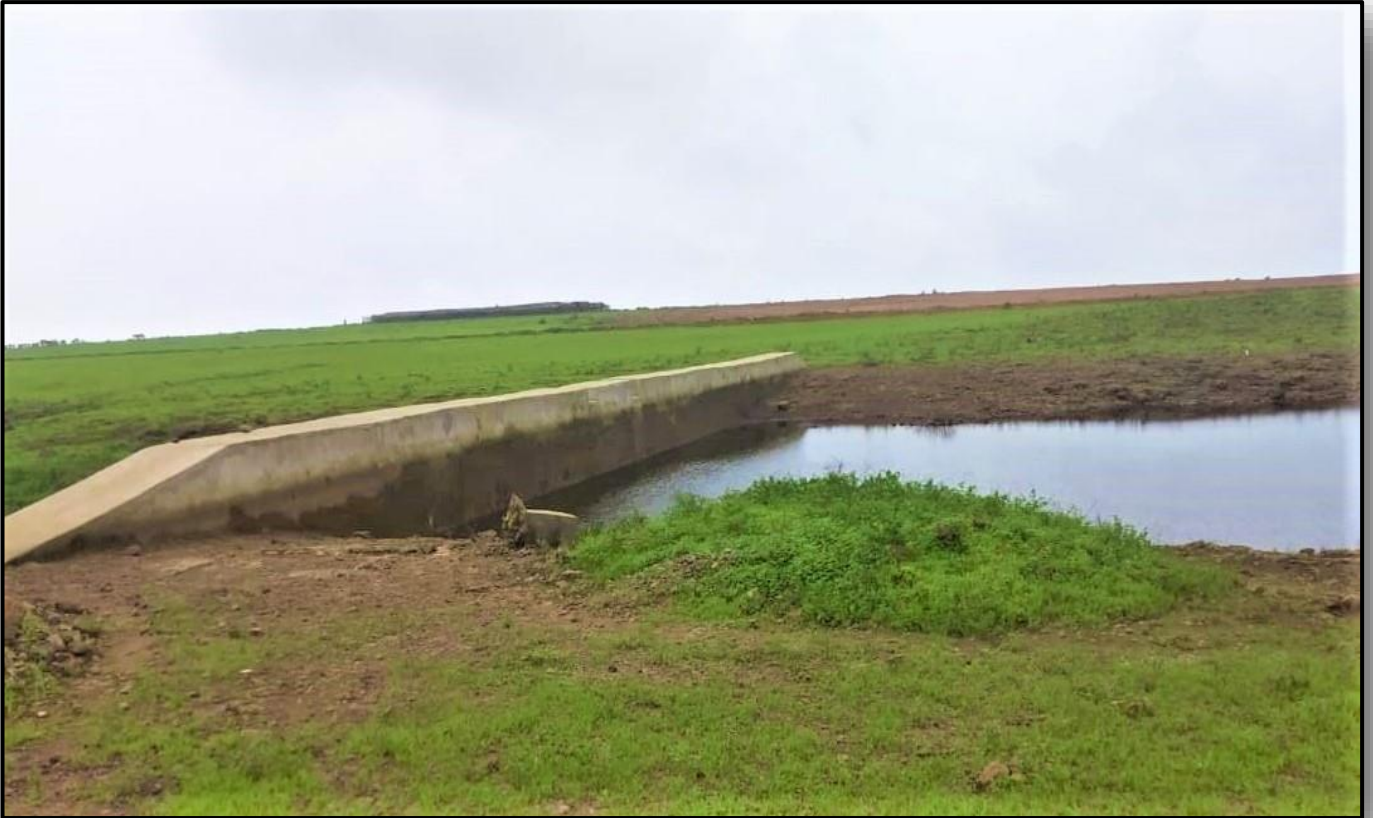
PHOTO 1: Showing Check dam
