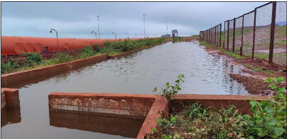
PHOTO 11: Surface Rainwater Harvesting Structure.
