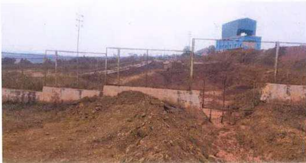
Figure 10: Fencing around the settling pit
