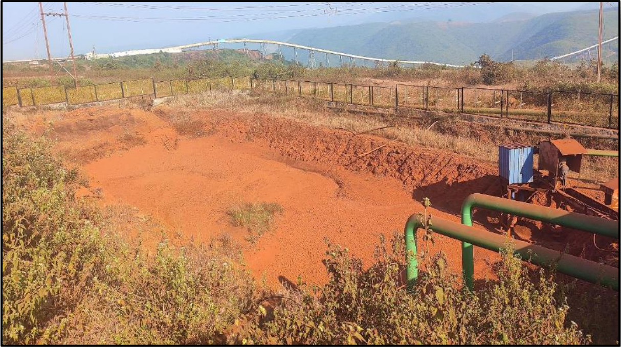
Settling Pit Near Crusher House
