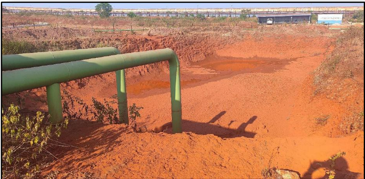
Settling Pond-1 Near Mines Entrance
