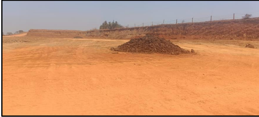
Land preparation for reclamation
