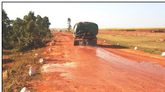
Water Sprinkling in the Haul Road
