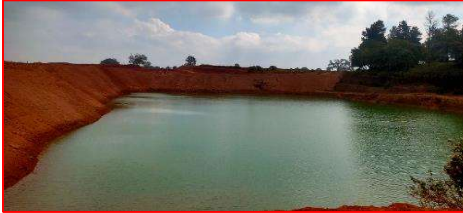
Rainwater Harvesting Pond
