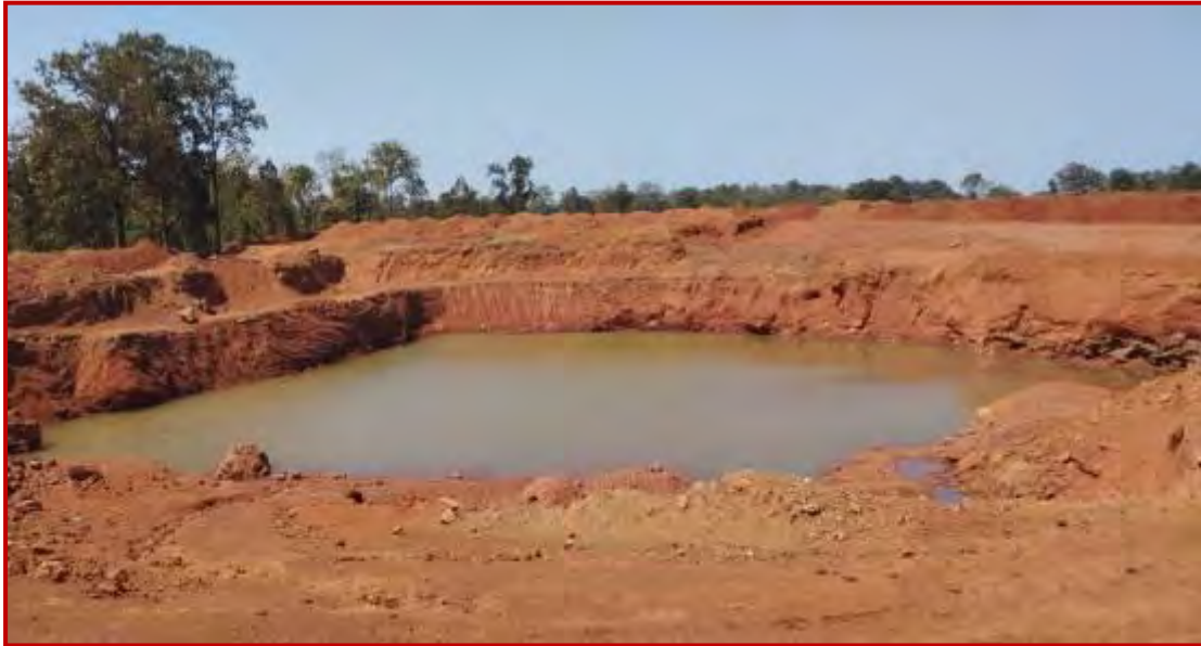
Rainwater Harvesting Pond
