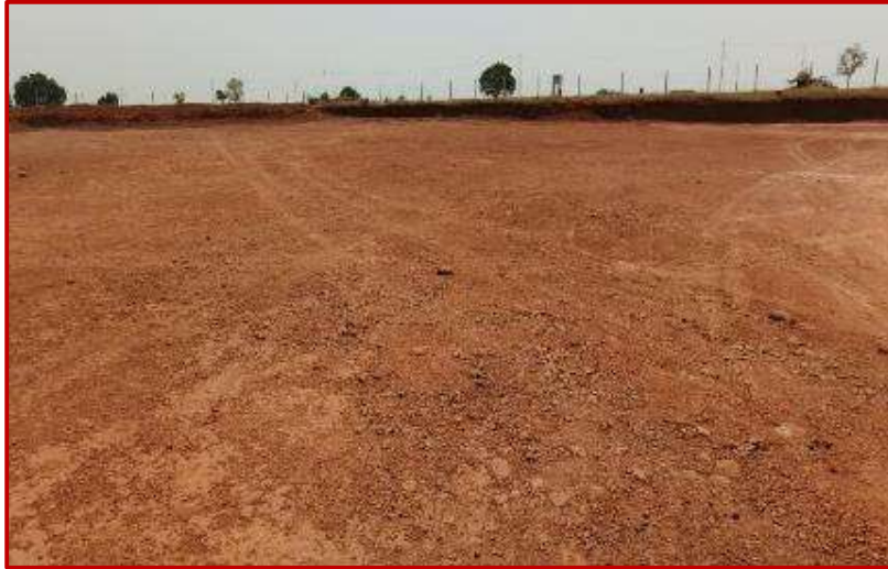
Reclamation of the mined-out area
