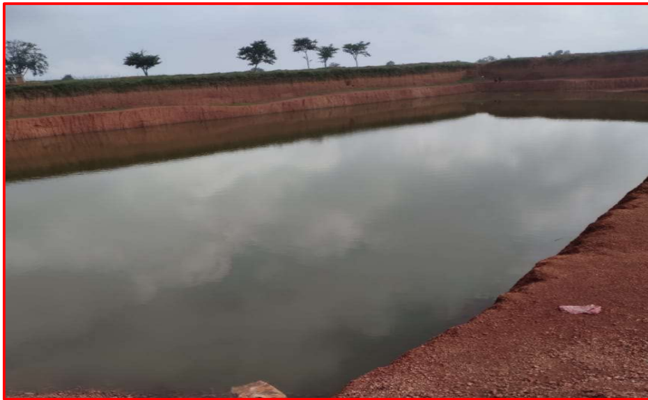
Rainwater Harvesting Pond
