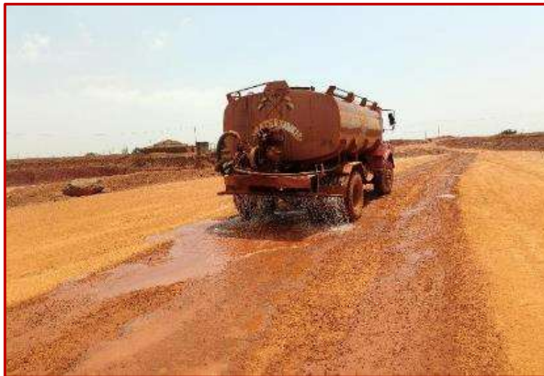
Water sprinkling through Tanker
