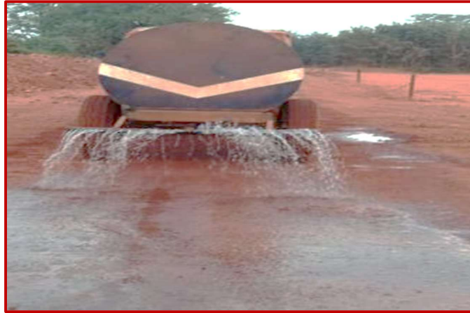
Water sprinkling through tanker.
