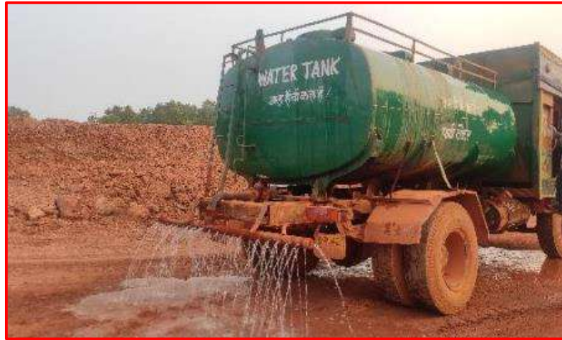
Water Sprinkling through Tanker
