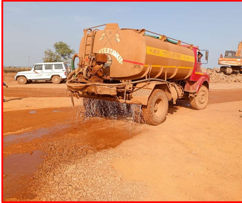
Water sprinkling through tanker
