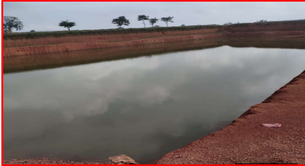
Rainwater Harvesting Pond
