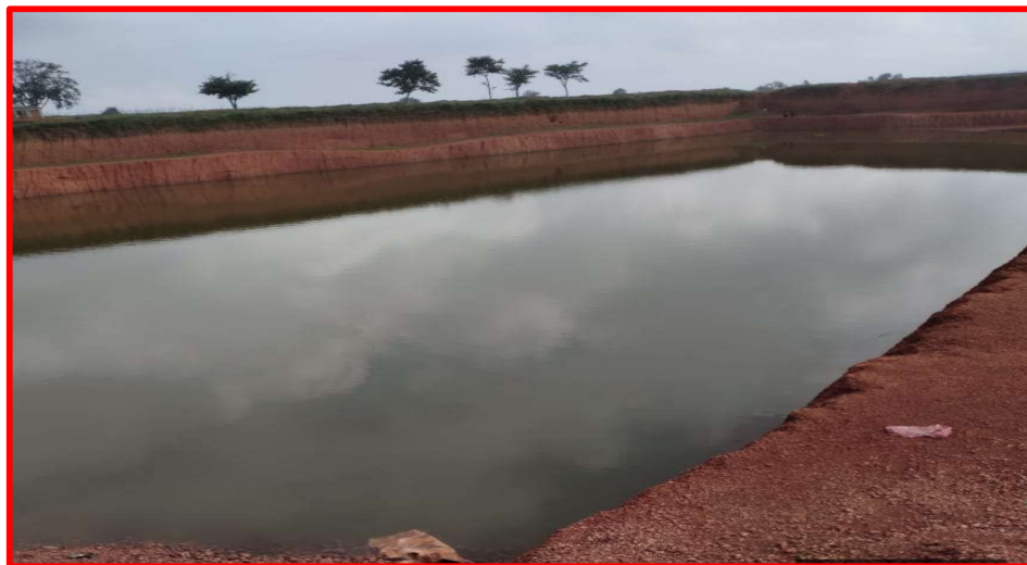
Rainwater Harvesting Pond
