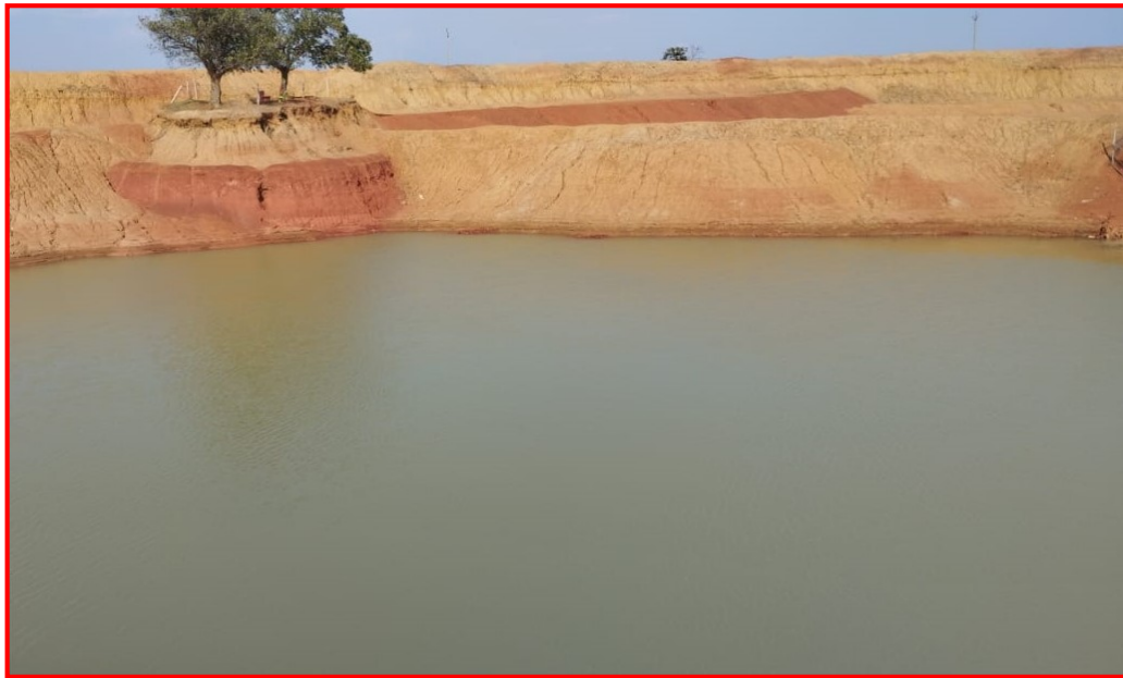
Rainwater Harvesting Pond with fencing.
