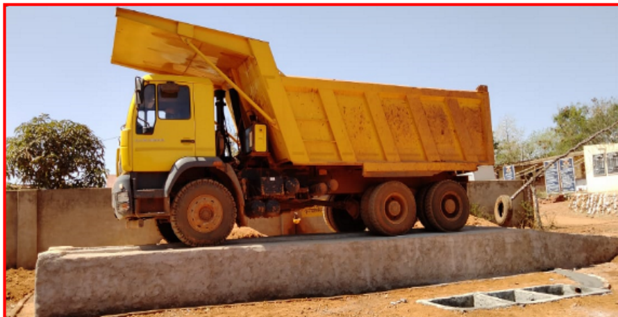
Washing Ramp with Oil and Grease Trap
