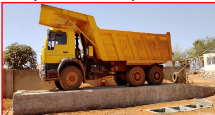
Washing Ramp with Oil and Grease Trap
