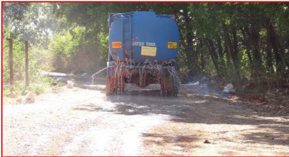
Water Tanker used for dust suppression
