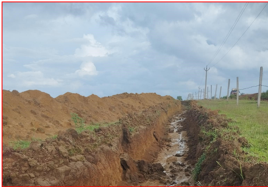
Garland drains around mine pit to prevent runoff.
