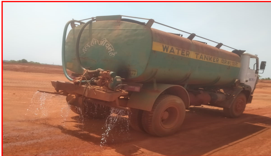
Water Sprinkling for dust suppression.
