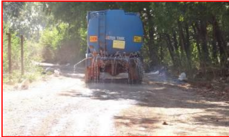
Water Sprinkling on Haul Road
