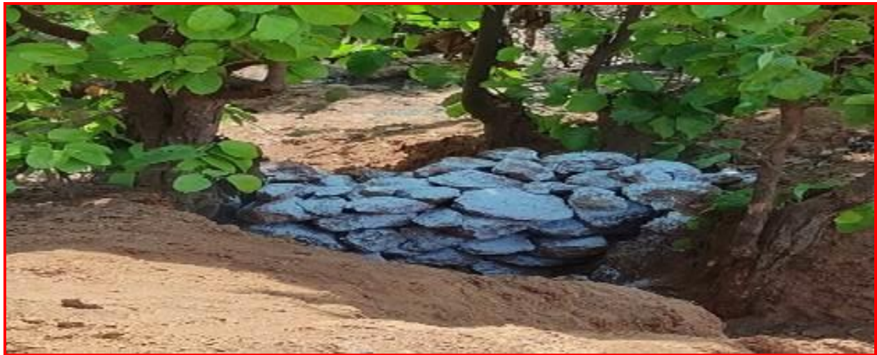
Retaining wall to prevent solid wash-off.
