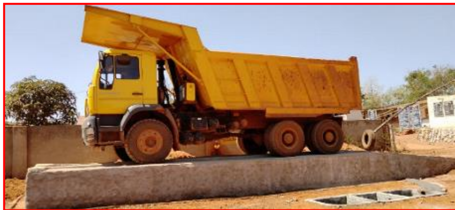
Washing ramp with Oil and Grease Trap
