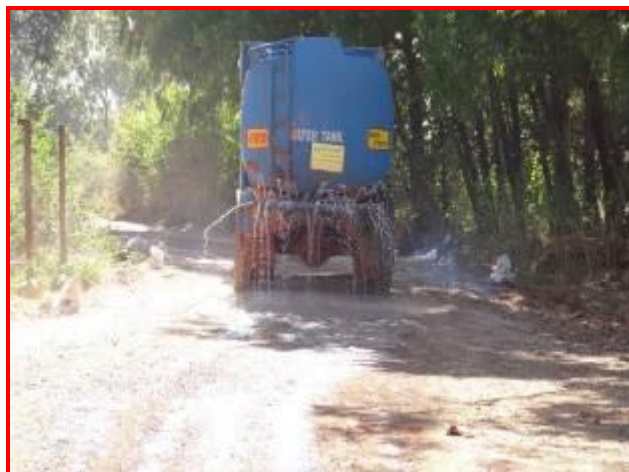
Water Sprinkling on Haul Road
