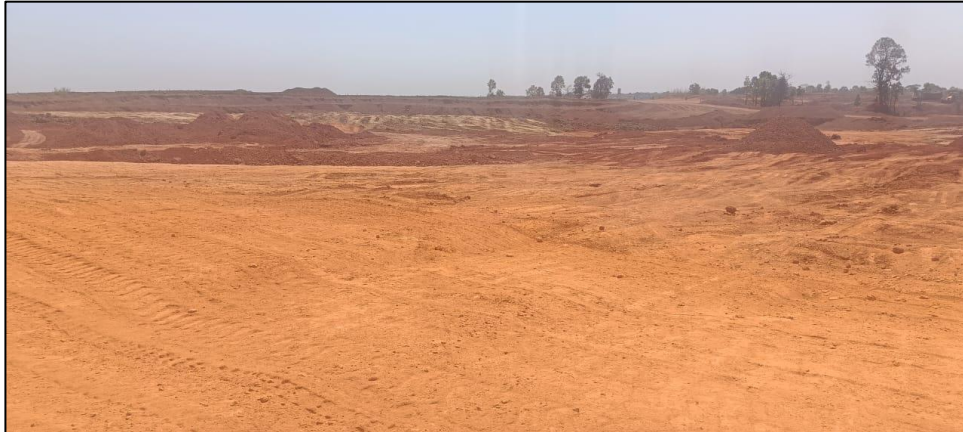
Top Soil Spreading for Backfilling
