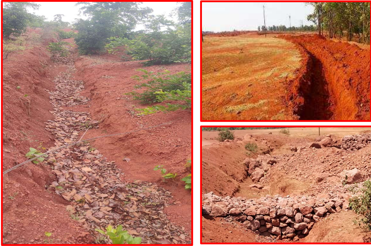
Garland drains & Siltation Pond
