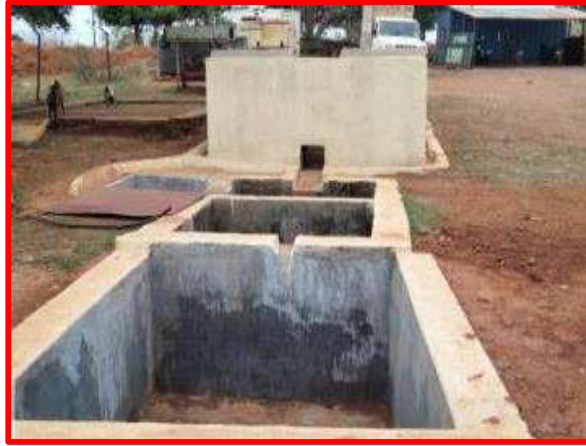
Washing Ramp and Oil and Grease Trap
