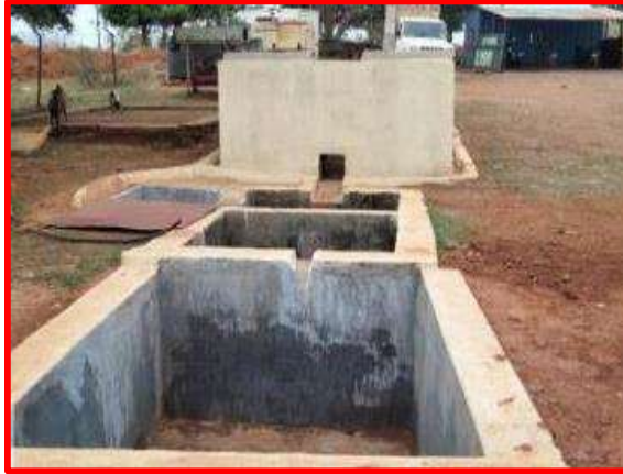
Washing Ramp and Oil and Grease Trap
