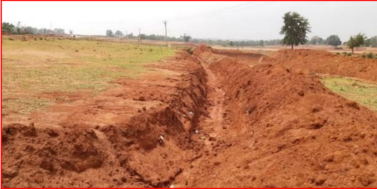
Garland drain around mine pit.
