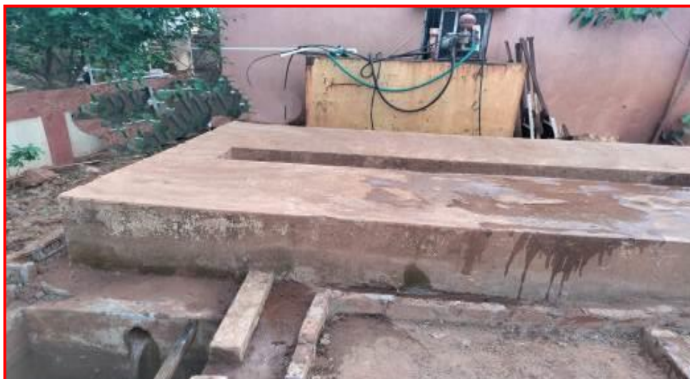
Washing Ramp with Oil and Grease trap
