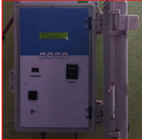
Piezometer Installed at Mine
