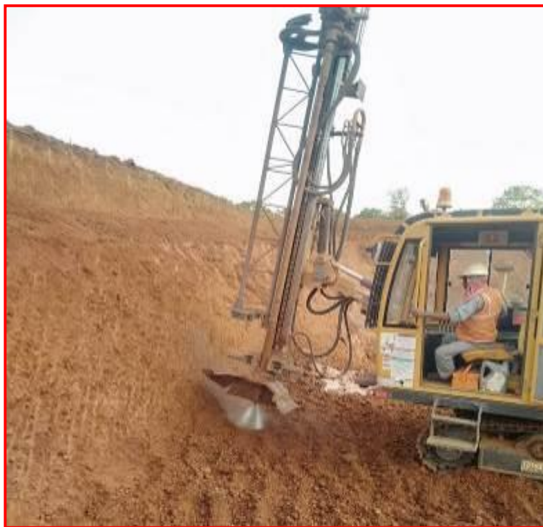
Wet drilling is being carried out.
