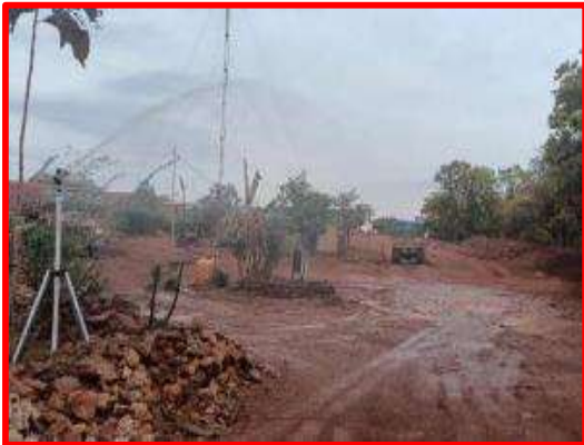
Installation of Fixed Type Water Sprinkler
