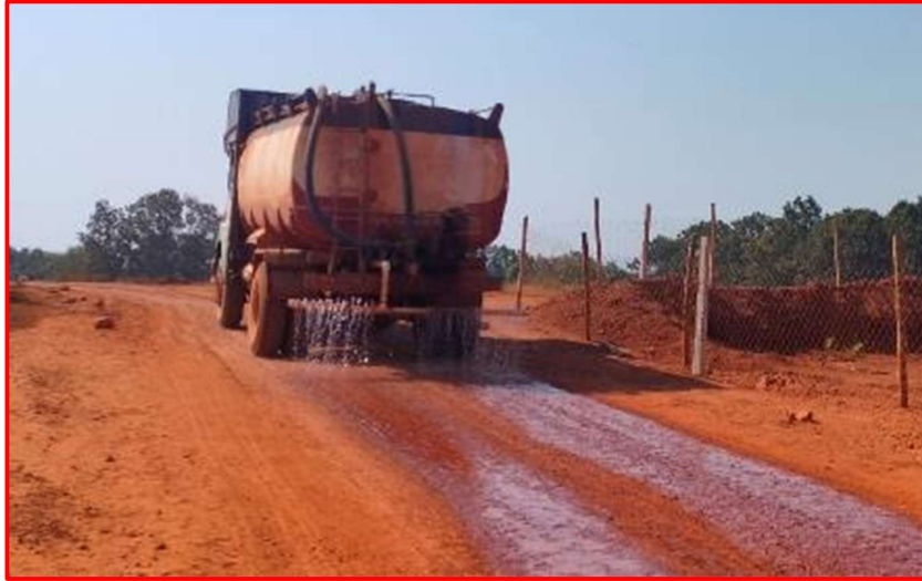
Sprinkling of water on roads
