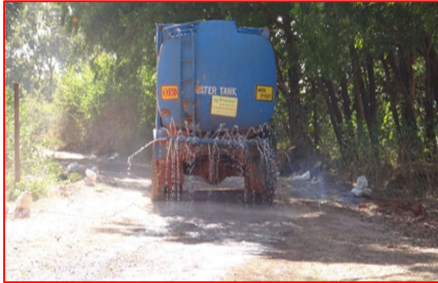
Dust suppression through water tanker.
