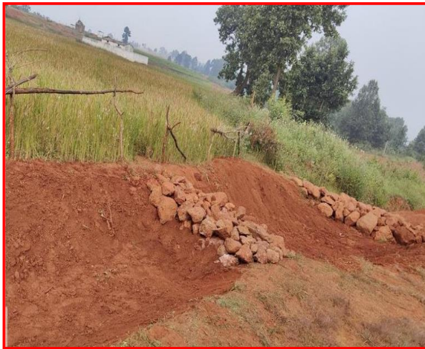
Retaining wall and siltation pit to prevent solid wash-off.
