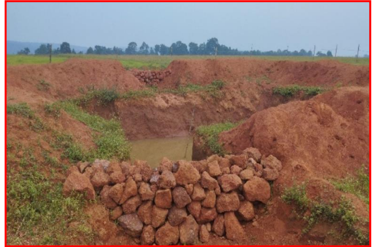
Retaining wall and siltation pit to prevent solid wash-off.
