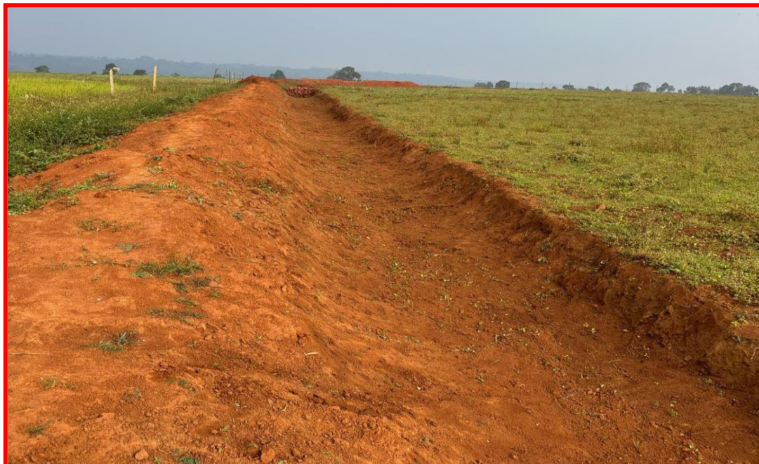
Garland drains around Mine pit.
