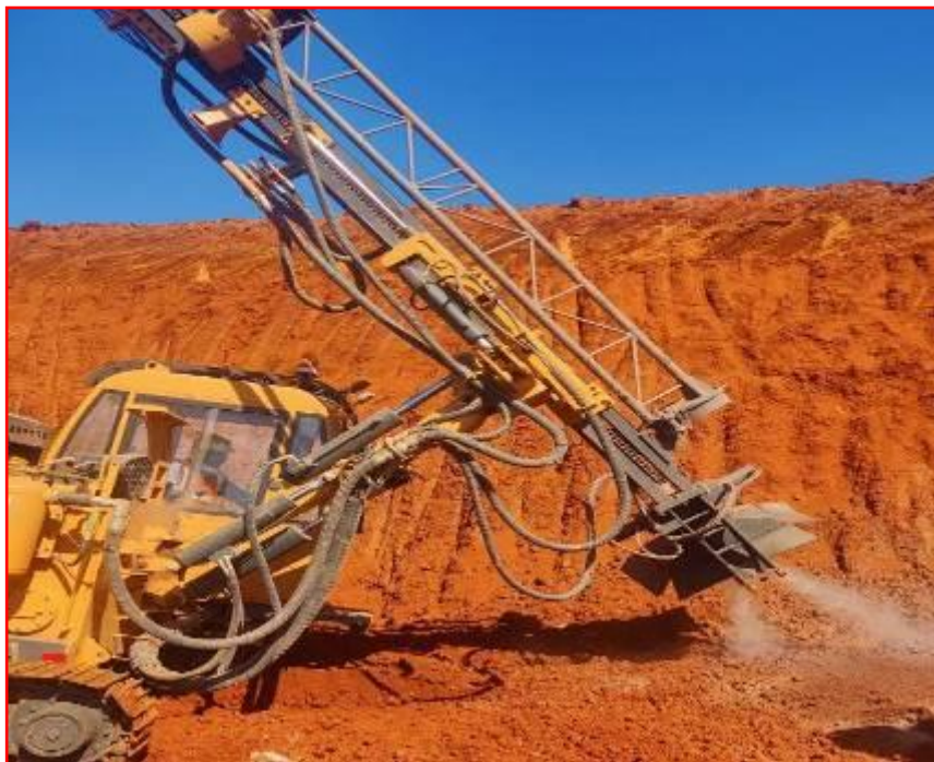
Wet drilling is in practice.
