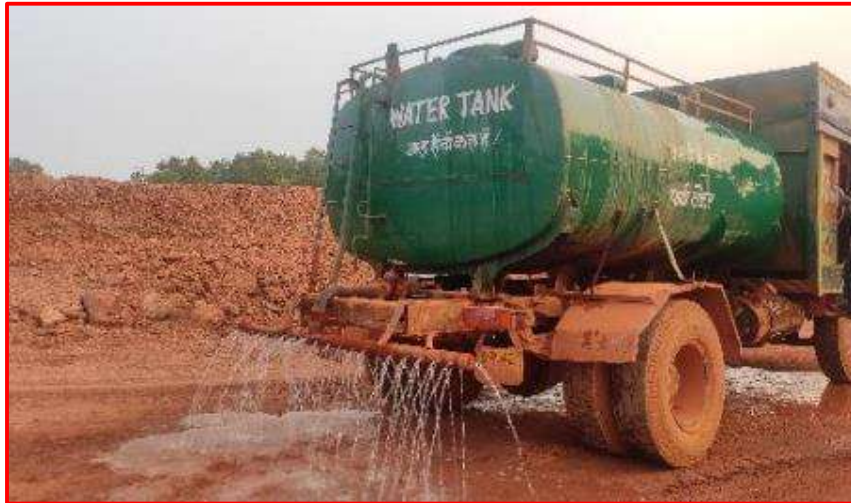
Dust suppression through water tanker.
