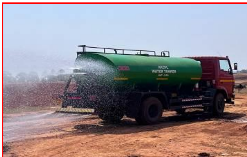
Water Sprinkling for Dust suppression.
