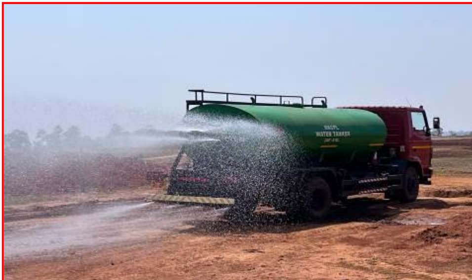
Water Sprinkling for Dust suppression.
