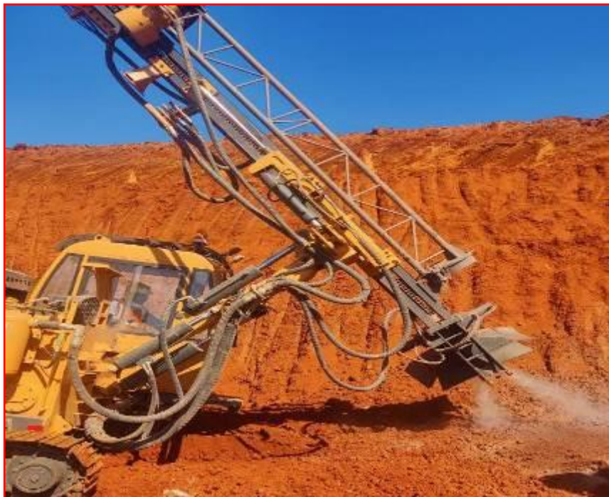
Wet drilling is in practice.
