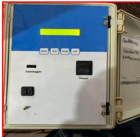
Piezometer Installed at Mine
