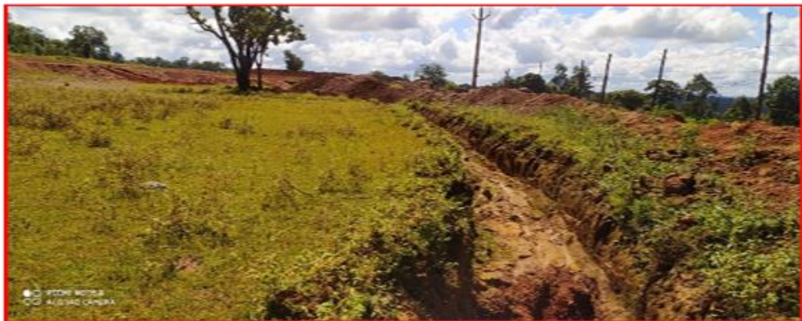
Garland drains around mine pit.
