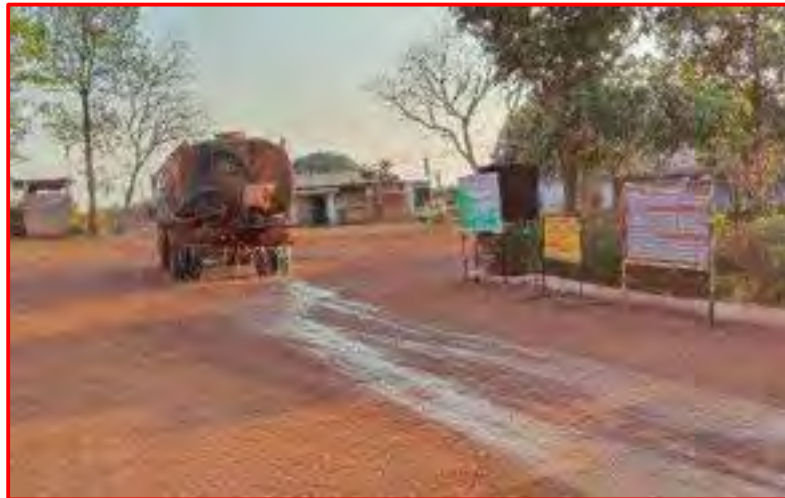
Water sprinkling through tanker
