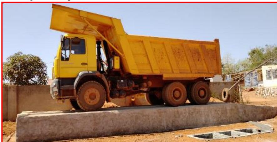
Washing Ramp with Oil and Grease Trap
