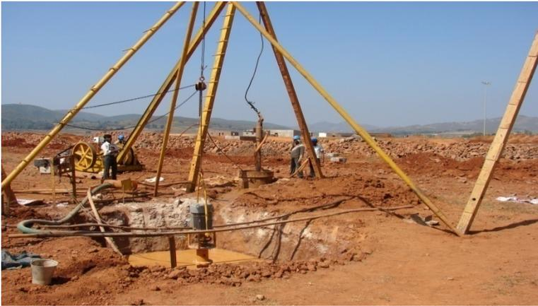
**CPP area: Piling work commenced in boiler and coal bunker area (M/s Rammana Rao & associates)**
