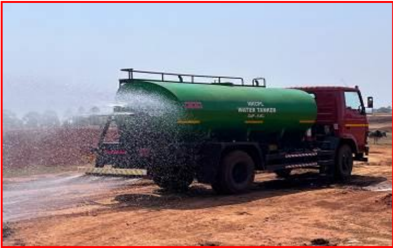
Water Sprinkling for Dust suppression.
