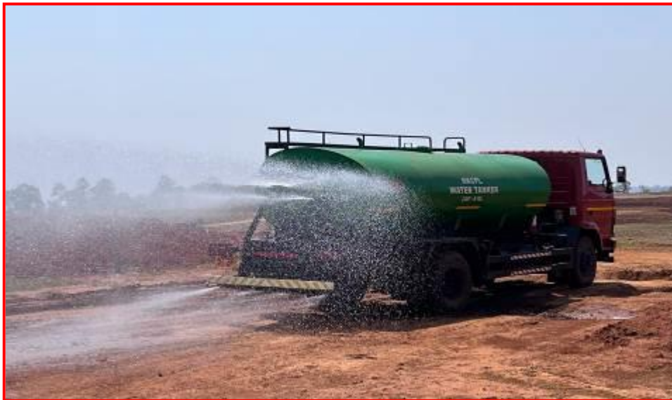
Water Sprinkling for Dust suppression.
