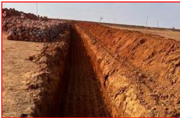
Garland drains around Mine Pit
