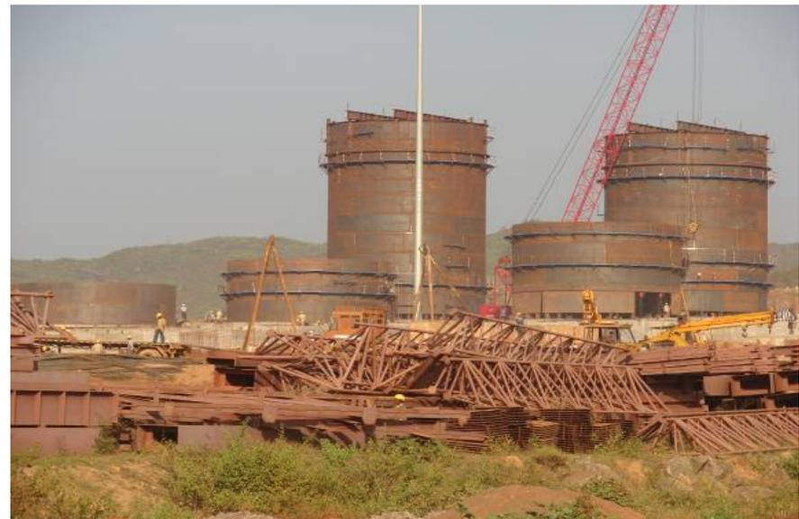
PPTs – 5 tanks shell erection in various stages (TK-202, 204, 205, 102 & 104)
