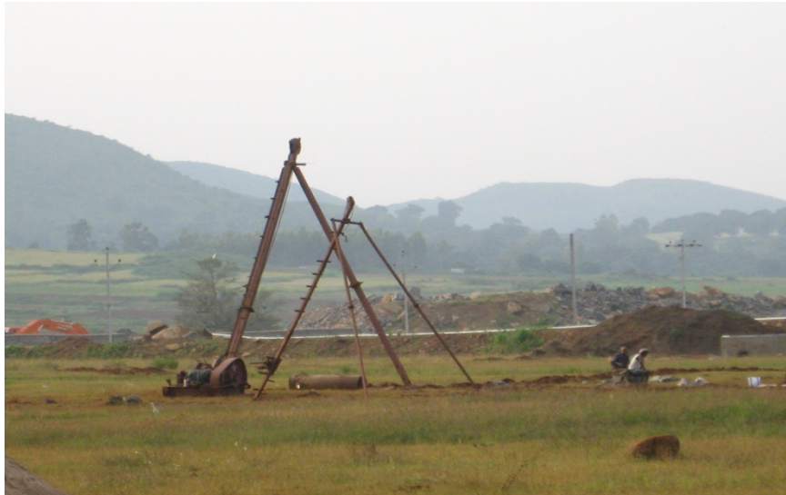
Non-plant buildings - Piling work commenced
