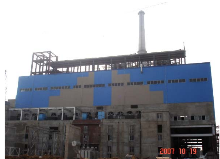
Power House structure Unit#4
