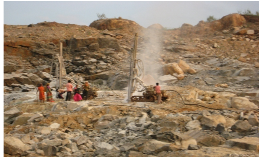
Hard rock cutting - drilling WIP
