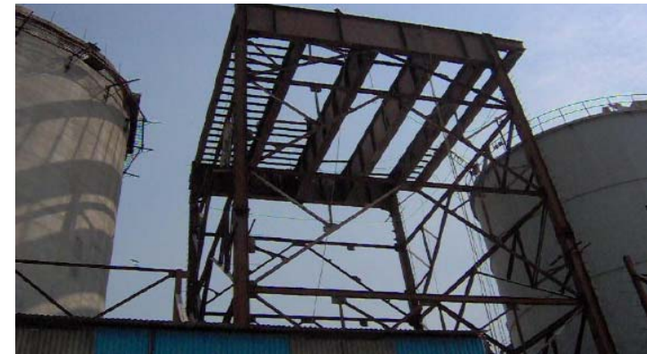
Structural erection of Alumina unloading system
