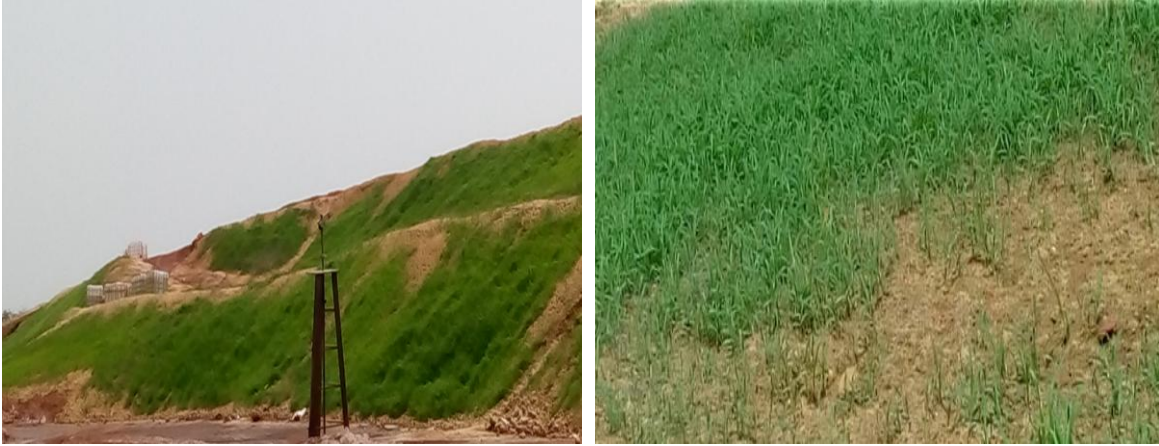
Photo: Green belt development in RMP by hydro-seeding technology
