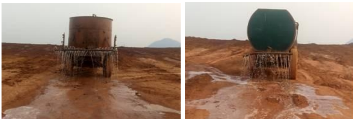
Photo: Dedicated water tanker in RMP area and road to suppress dust
