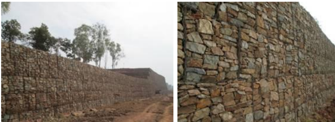
Photo: Gabion & Reinforced Soil Wall
