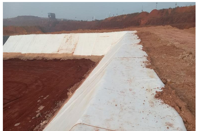
Backfilling of mine void at Baphlimali
