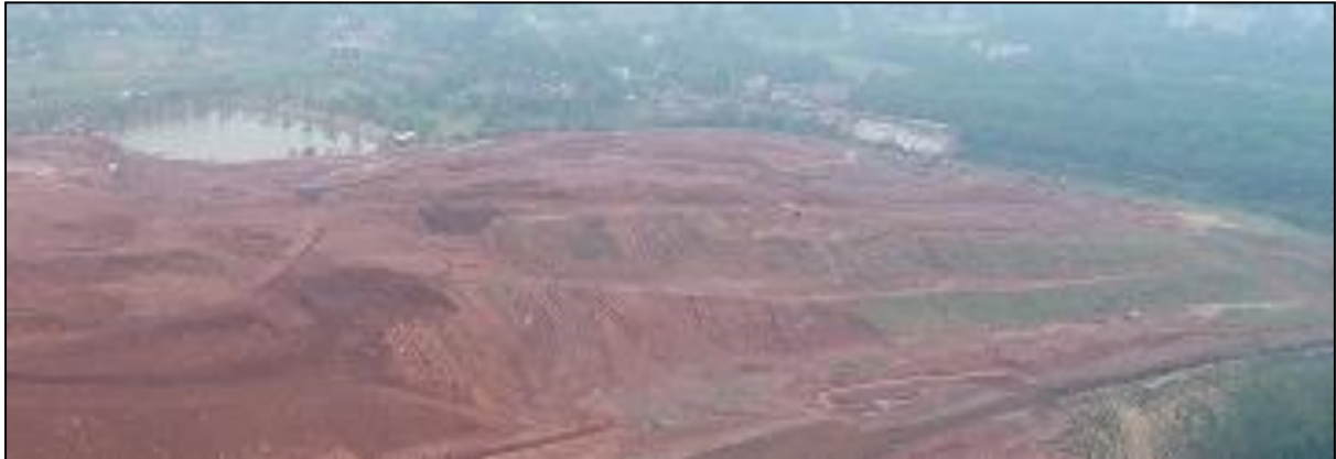
RMP 3 & 4 : Before rehabilitation project at Muri
