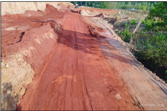
Pilot project of Road construction using Red Mud near Koraput
