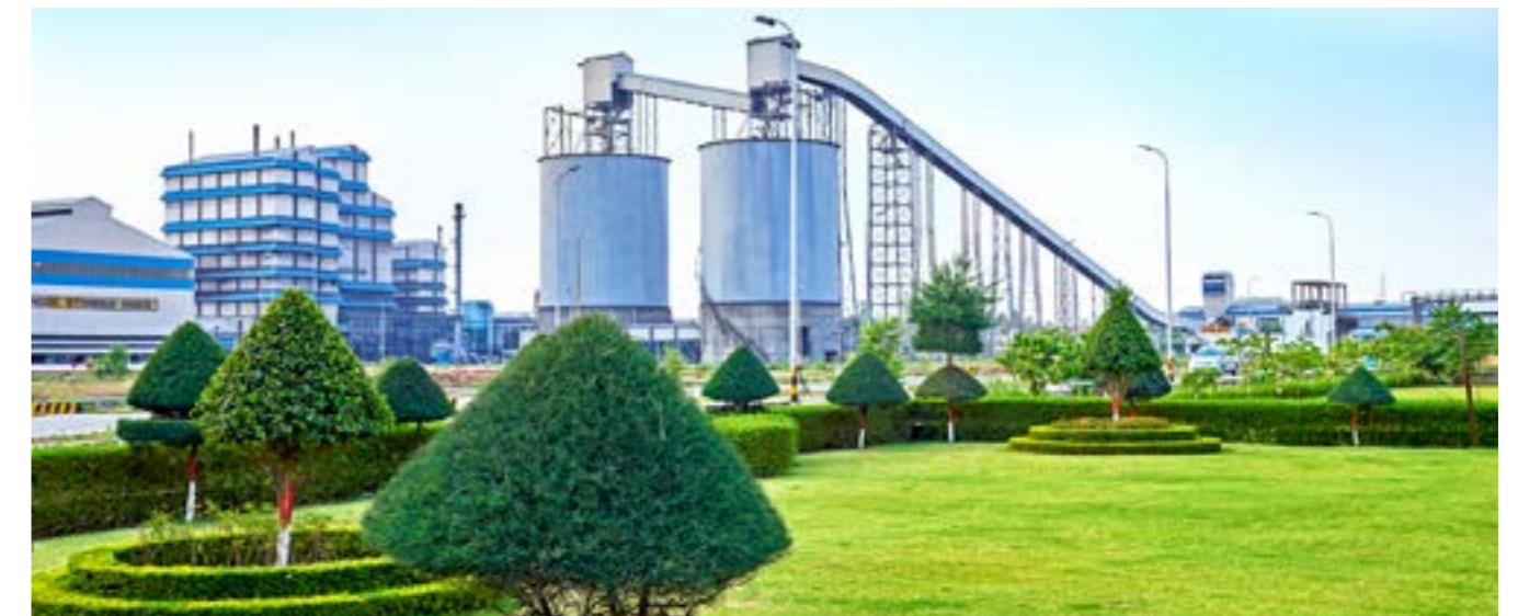
A view of the Mahan Smelter, The plant was conferred Mission Energy's 'Best Energy Efficient' Plant in coal preparation category (2021)
