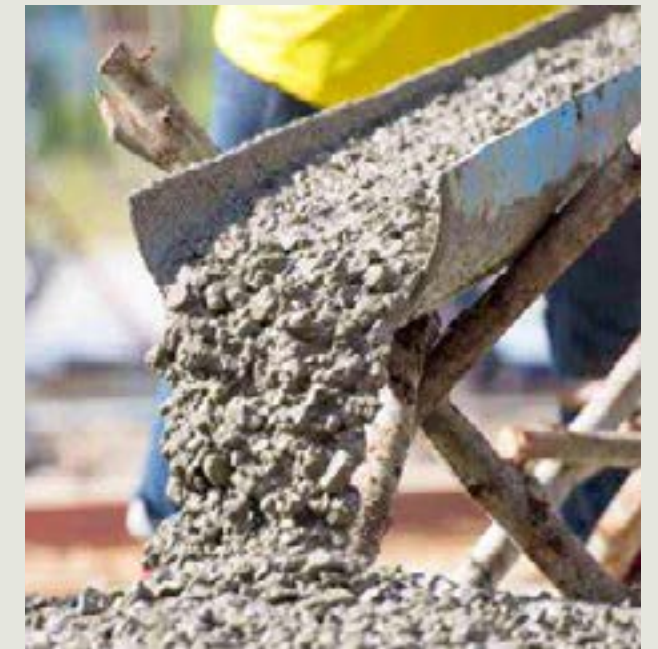
Copper slag is being used to replace sand in concrete
